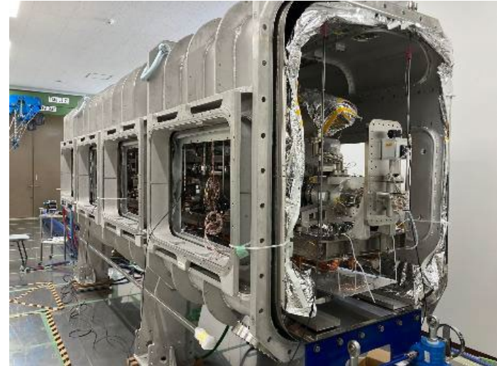
Insertion of cold mass into the cryomodule
